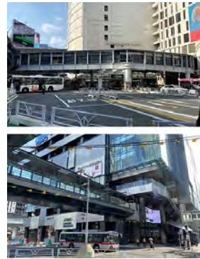
(Top) Shibunishi Deck (Bottom) SHIBUYA FUKURAS Connection Deck
