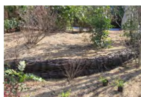
4.Earth retaining Natural material earth retaining
