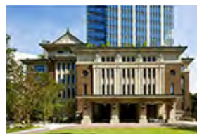
Exterior of Kudan-Kaikan Terrace (preserved area)
