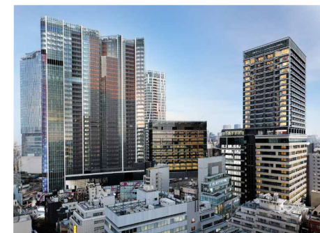
Shibuya Sakura Stage, completed in November 2023
