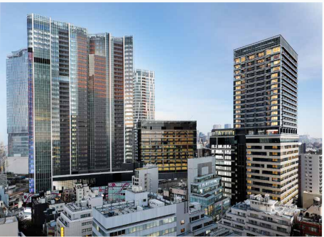
Shibuya Sakura Stage, completed in November 2023
