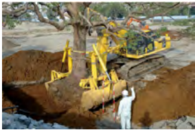
Transplanting work using a TPM machine
