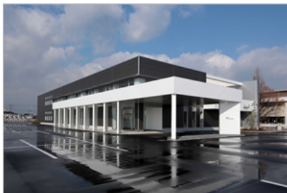
Yonago Operation Center (Yonago City, Tottori Prefecture)
