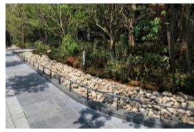
2.Disaster prevention and mitigation Rain garden
