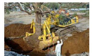
Transplanting work using a TPM machine
