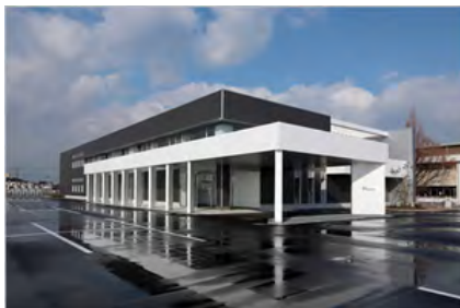
Yonago Operation Center (Yonago City, Tottori Prefecture)
