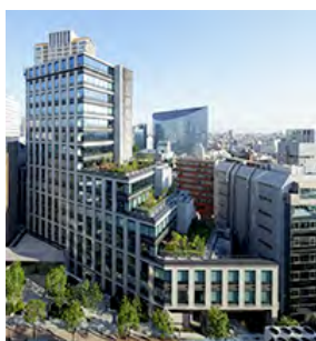
Shin-Meguro Tokyu Building
