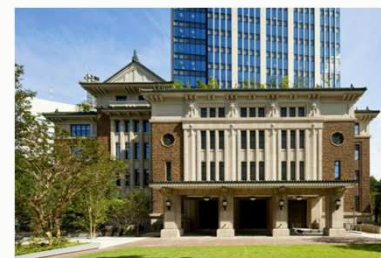
Exterior of Kudan-Kaikan Terrace (preserved area)
