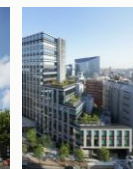
Shin-Meguro Tokyu Building
