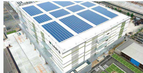
ReENE LOGI'Q Kyoto Kumiyama Solar Power Plant
