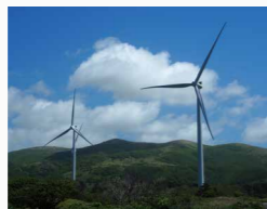
ReENE Matsumae Wind Power Plant
