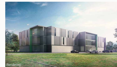
The exterior of the data center
