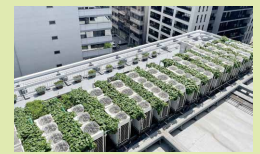
The Unosawa Tokyu Building's potato-based greening system
