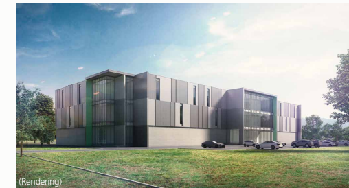
The exterior of the data center
