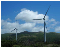
ReENE Matsumae Wind Power Plant
