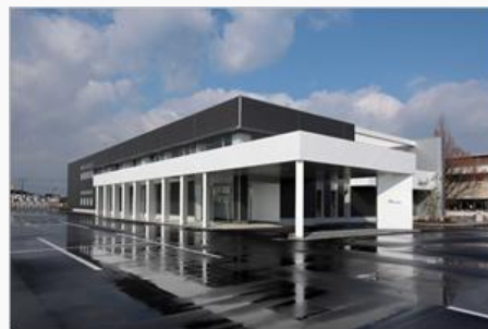
Yonago Operation Center (Yonago City, Tottori Prefecture)
