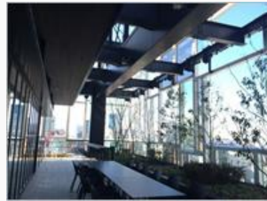
Eave materials for the Shin Aoyama Tokyu Building
