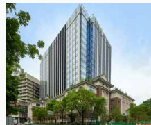
Plans for Kudan-Kaikai Terrace (completed in July 2022) acquired a five-star rating under the DBJ Green Building Development Plan Certification program
