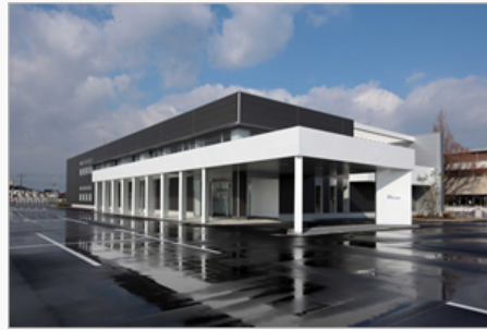
Yonago Operation Center (Yonago City, Tottori Prefecture)
