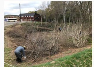
Cleaning the pond
