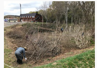
Cleaning the pond
