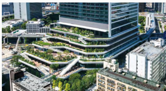
TOKYO PORTCITY TAKESHIBA (Completion: May 2020)
