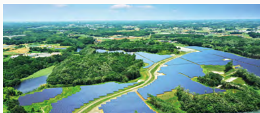
ReENE Namegata Solar Power Plant (Commencement of operation: October 2020)
