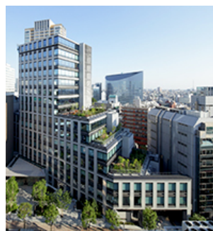
Shin-Meguro Tokyu Building
