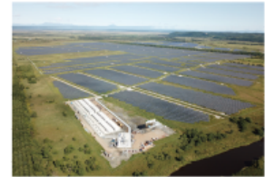
Suzuran Kushirocho Solar Power Plant
