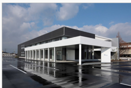
Yonago Operation Center (Yonago City, Tottori Prefecture)
