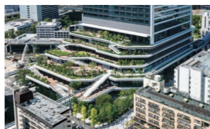
The office tower and residence tower cover a combined area of around 200,000m 2 . The office tower is home to a variety of tenants, including the Tokyo Metropolitan Industrial Trade Center.
