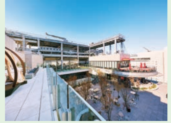
SHIBU NIWA, a rooftop garden on the 17th floor that commands a panoramic view of Shibuya
