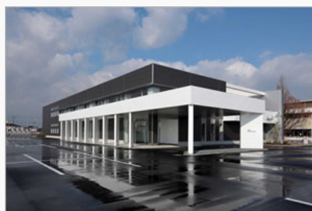
Yonago Operation Center (Yonago City, Tottori Prefecture)
