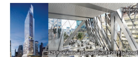
425 Park Avenue (Completion: FY2019 (Planned))
