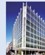
Nihombashi Honcho Tokyu Building Location: Chuo-ku, Tokyo Completion: October 2004
