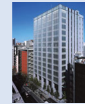
Shibuya Minami Tokyu Building Location: Shibuya-ku, Tokyo Completion: January 2005
