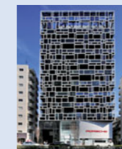
Shin-Aoyama Tokyu Building Location: Minato-ku, Tokyo Completion: January 2015
