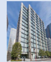
Uchisaiwaicho Tokyu Building Location: Chiyoda-ku, Tokyo Completion: July 2006
