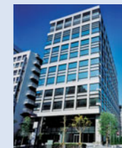
Ichigaya Tokyu Building Location: Chiyoda-ku, Tokyo Completion: October 2004
