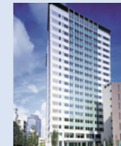
Ebisu Business Tower Location: Shibuya-ku, Tokyo Completion: November 2003
