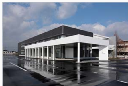
Yonago Operation Center (Yonago City, Tottori Prefecture)
