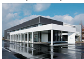
Yonago Operations Center (Yonago City, Tottori Prefecture)
