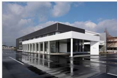
Yonago Operation Center (Yonago City, Tottori Prefecture)
