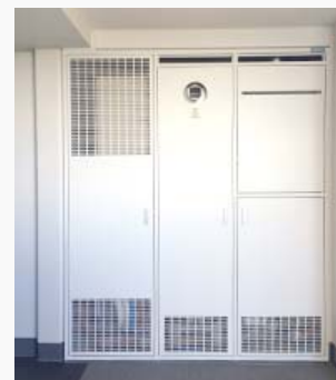
Enefarm for condominiums
