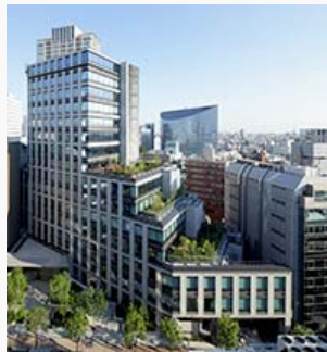
Shin-Meguro Tokyu Building
