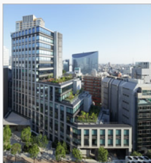
Shin-Meguro Tokyu Building
