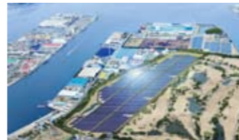
Mega solar project in Kagawa Prefecture
