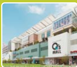
Commercial facilities suited to their communities
