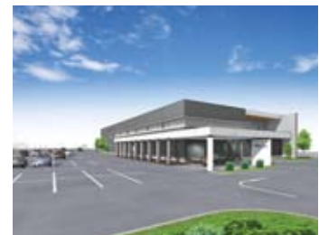
Yonago Operation Center (tentative name)
