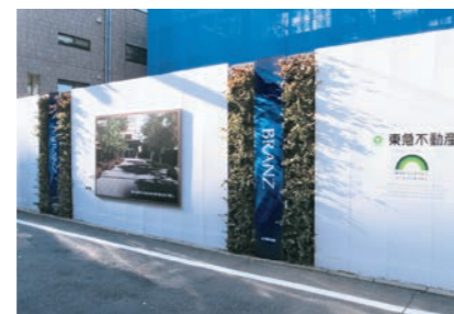
Greening of the temporary fence at a construction site
