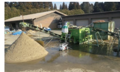
Bunker sand washing system
