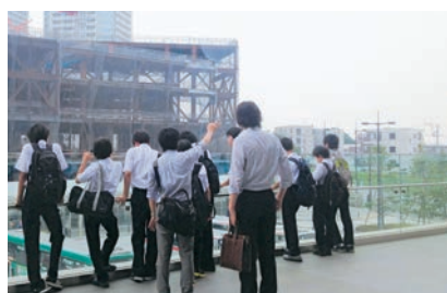
Local junior high school students visited a construction site
