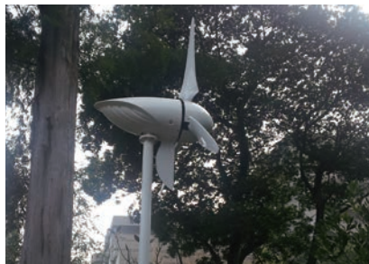
Wind turbine installed within the premises of Tokyu Harvest Club Atami Izusan & VIALA
