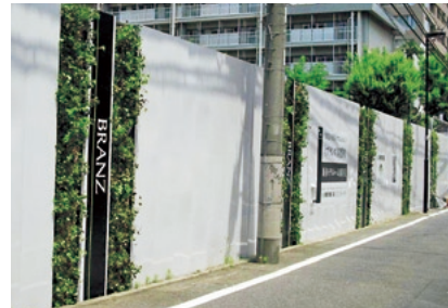
Temporary enclosure with greenery (BRANZ Yonbancho)
