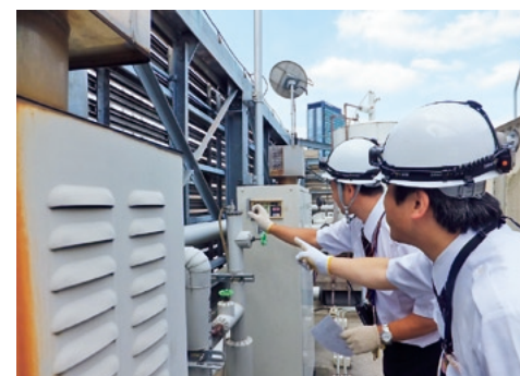
Disaster response training (Tokyu Relocation Co., Ltd.)
