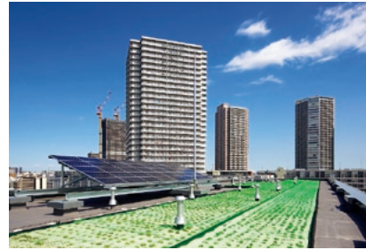
Green roof and solar power generation equipment at the BRANZ Shinonome
