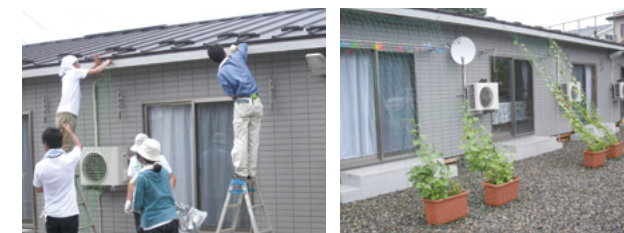
Installation of green curtains
