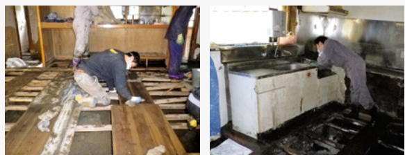
Cleaning mud out of a house damaged by the tsunami/Cleanup work
