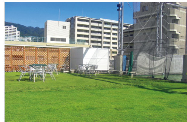
Green roof technique at Sumiyoshi branch of Tokyu Sports Oasis, Inc.
