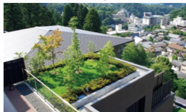
Green roof on Tokyu Harvest Club Arima Rokusai
