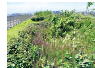
Green roof technique, "Picnic Turf"
