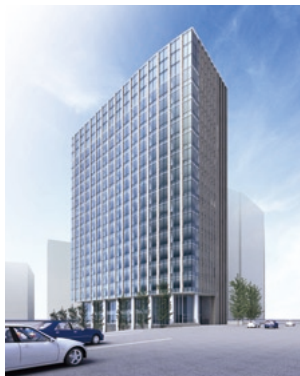
Kasumigaseki Tokyu Building
